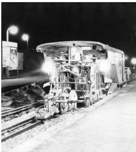
Tamping machine, Oxshott station, 25 March 1975 © Stephen Spark
