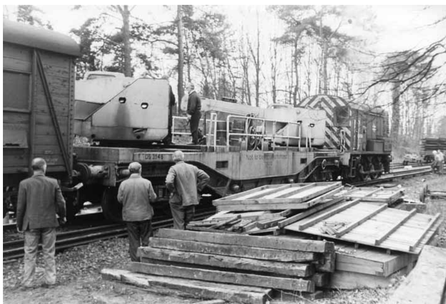
Track relaying crane, Oxshott, 24 March 1975 © Stephen Spark
